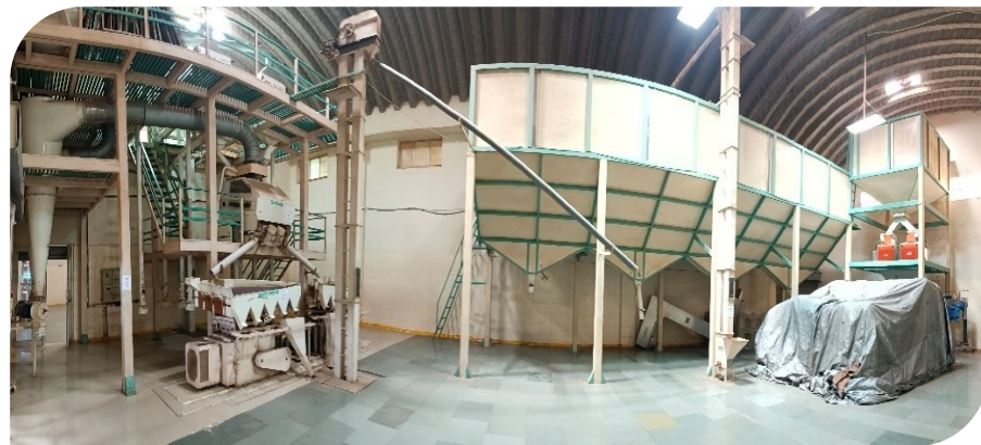
Navrang Cleaning Plant
